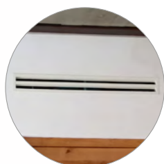
SLITTED LINEAR DIFFUSER
